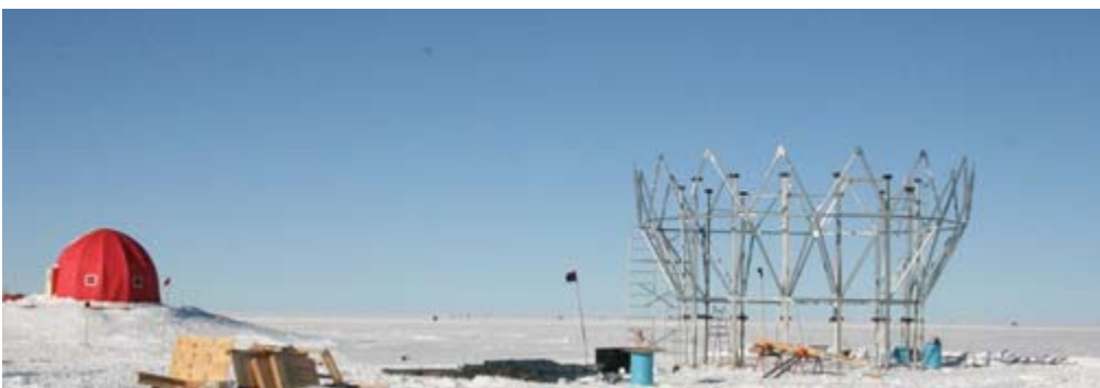
The dome structure grows
