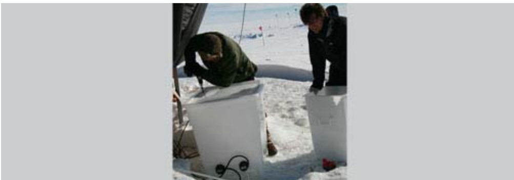
Cooks snowmelter under construction.
