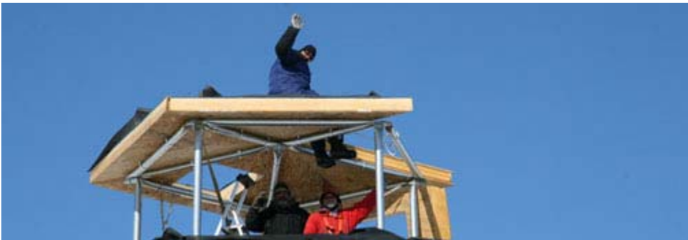
Zoom-in on the cupola roof builders in action.
