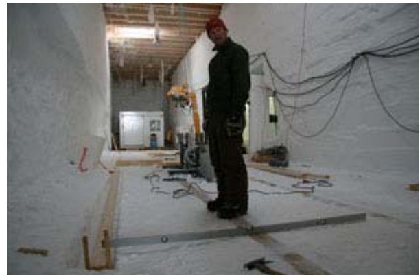
Floor constructions in the drill trench
