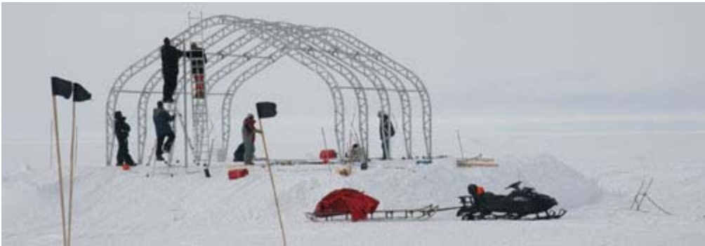
Building the second garage
