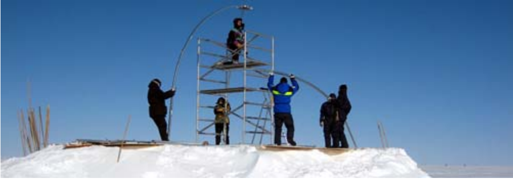
Afternoon constructions. The frame for a dome tent is assembled.
