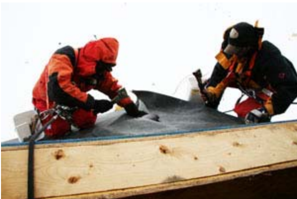
Fixing the rubber panels on the roof
