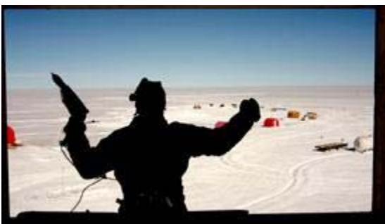
The hardworking rappelling team on the dome shell
