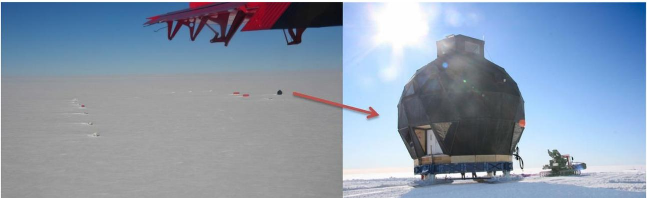
*Left: Fly over photo of the stored NEEM camp May 2013. The line to the left is sledges with equipment stored and the black building to the right is the main dome on skis. In the two red tents the tracked vehicles are stored. Right: Photo from 2011 of the 4 storey, 45 ton main dome on skis being pulled by the NEEM Pistenbully.*
