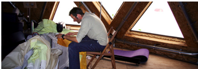
Tim repairing the outdoor toilet tents
