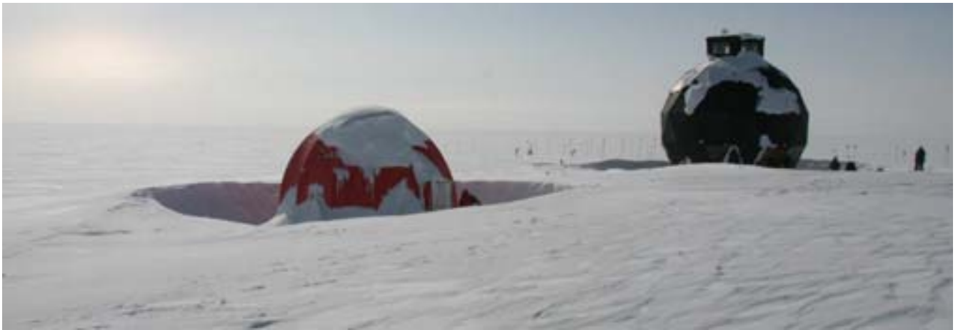
Red dome and main dome in snow drifts. It is hard to imagine that the red dome was built on a 2 m snow hill two years ago. Note the person on the right for size comparison.
