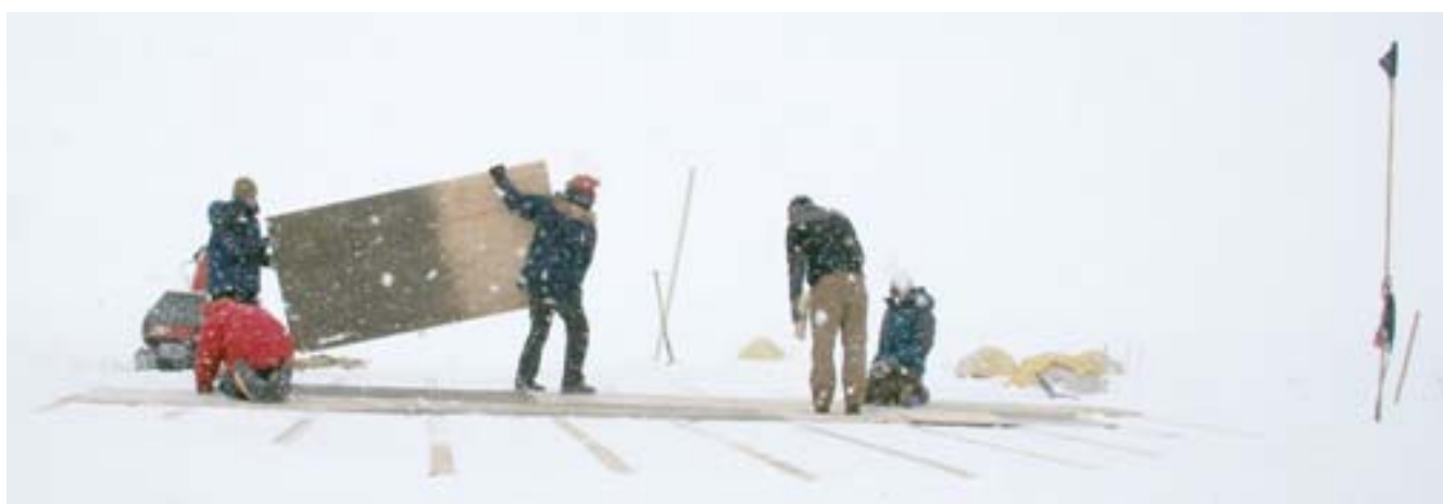
Floor is being laid for the red dome tent. The work was a little difficult due to snow. Christopher is hammering nails, Theo and Peter are carrying plywood, Sverrir knocks the sheets in place and Lou is nailing them.
