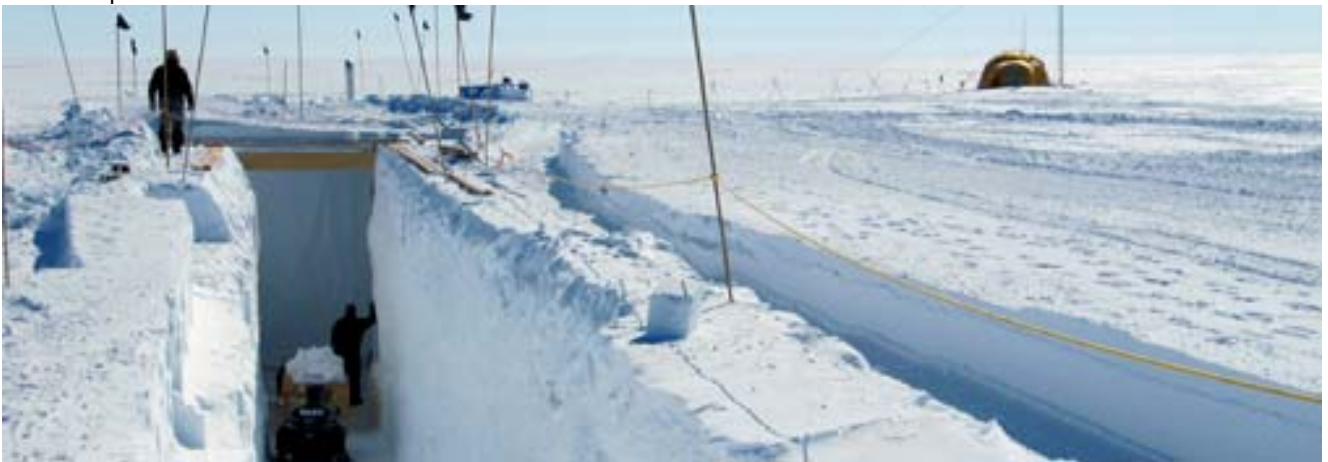
Excavation of trench for elevator and staircase.
