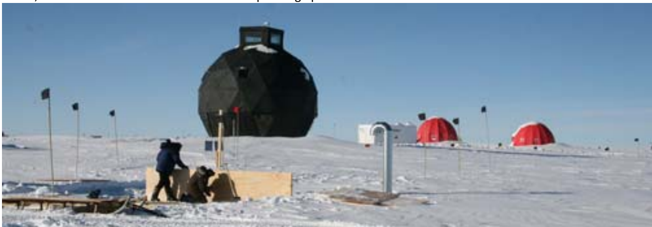
Mounting of the skylight with the main dome in the background.
