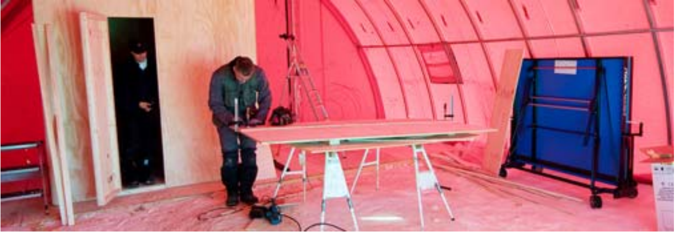
Construction of the sauna by Alli and Aksel.
