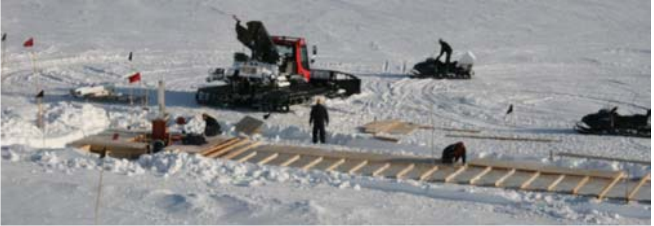
A scene from laying roof on the elevator trench..
