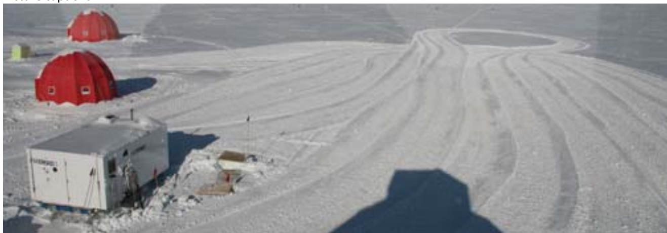
Removing snowdrifts around generator and main dome.
