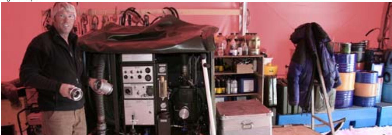
Sverrir in the mechanical garage with the fittings for the backup fuel station.
