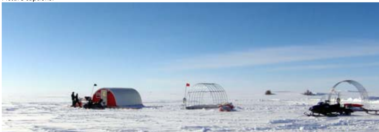
Building the last weatherports.
