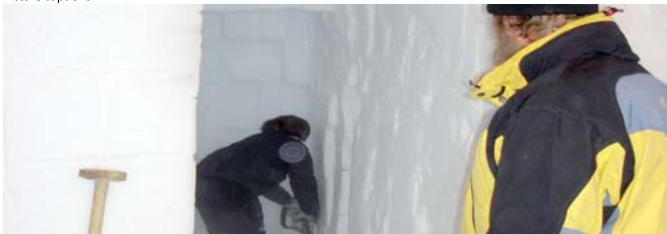
Maggan excavates cooling tunnel.
