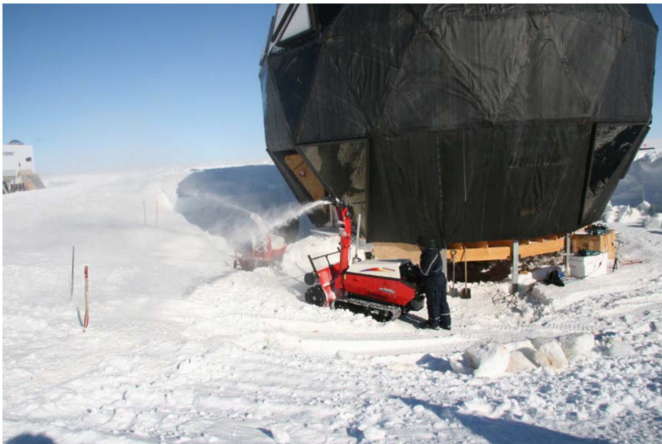
Using snow blowers to remove snow around the Dome
