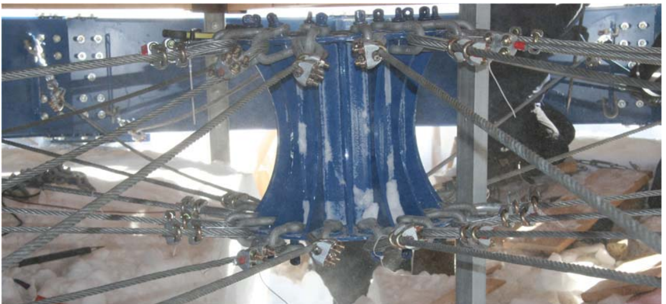
Centre axle for the 'bicycle wheel' under the Dome
