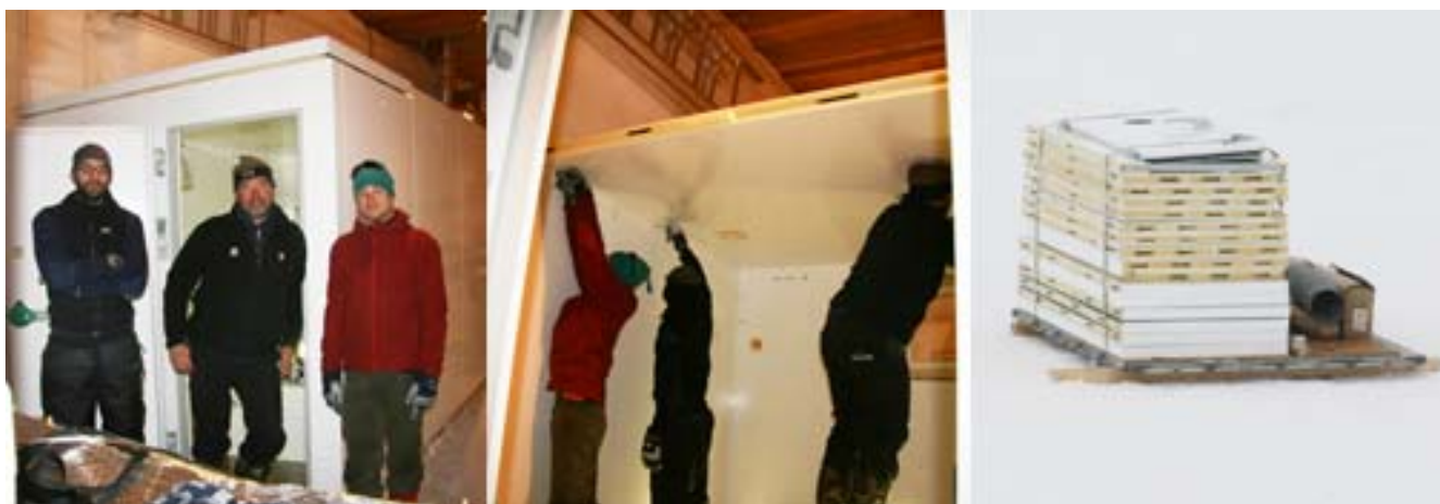
Disassembling and palletizing the GIL Viessmann cabin: Before, during and after
