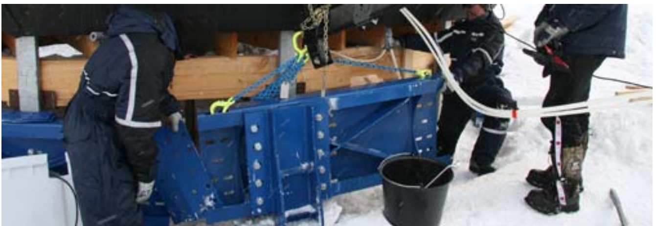
Placing the first of the 15 panels forming the Dome ring
