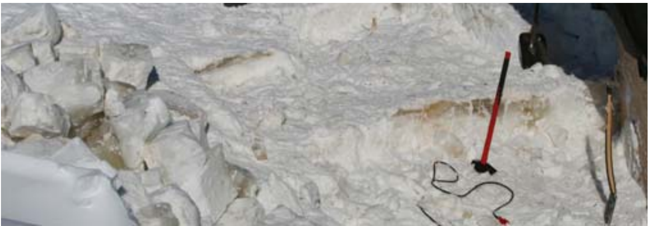
Chopping ice around the main Dome in order to free the 15 legs
