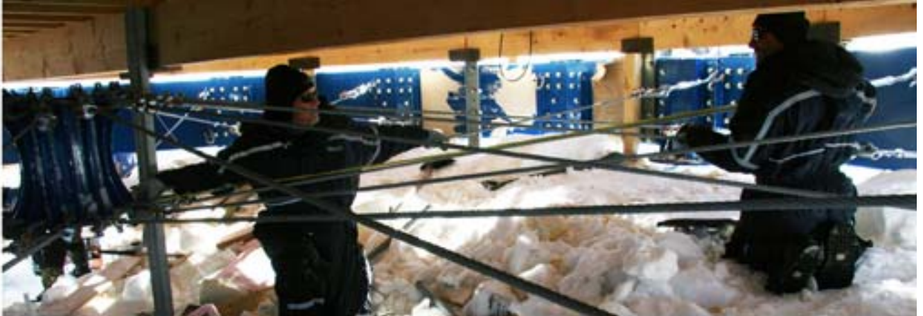
Mounting the cables onto the blue ring under the Dome
