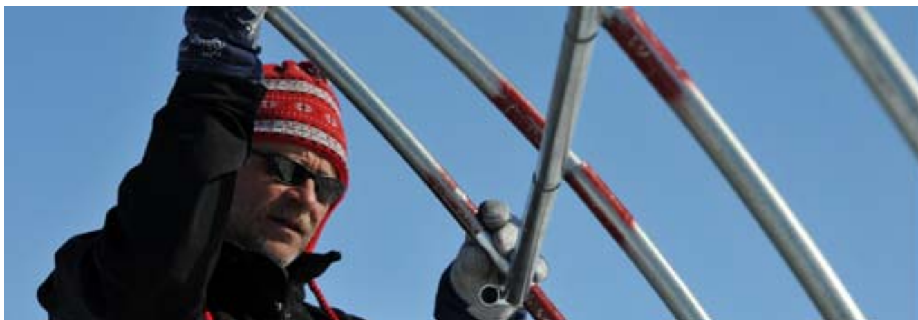
HansChr: Hans Christian is assembling the frame for a weatherport.
