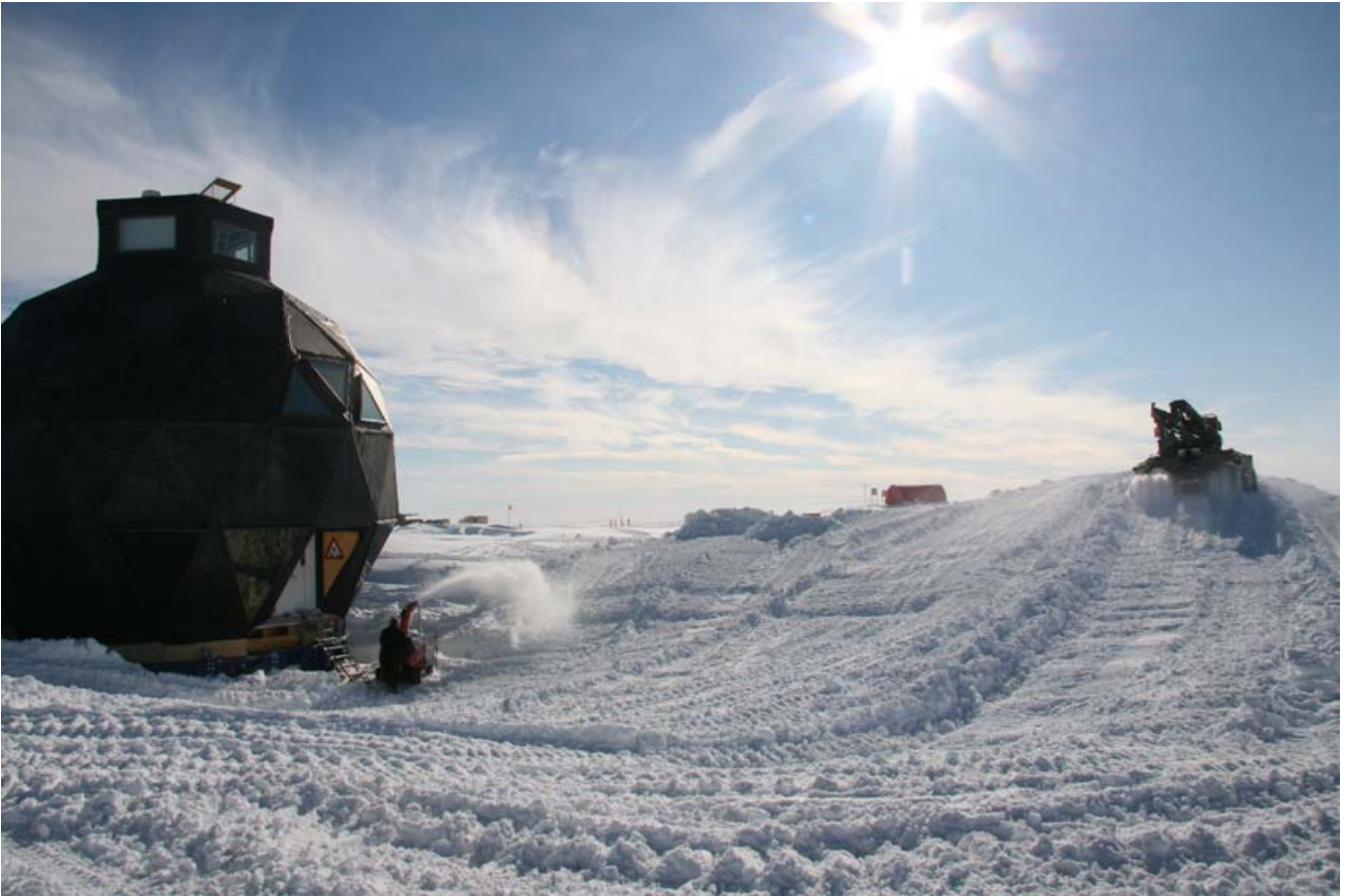
Preparing the ramp for the dome move
