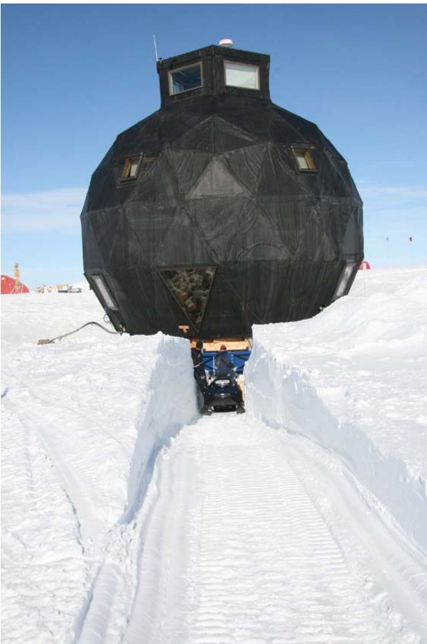
Trench to get the skies down under the frame
