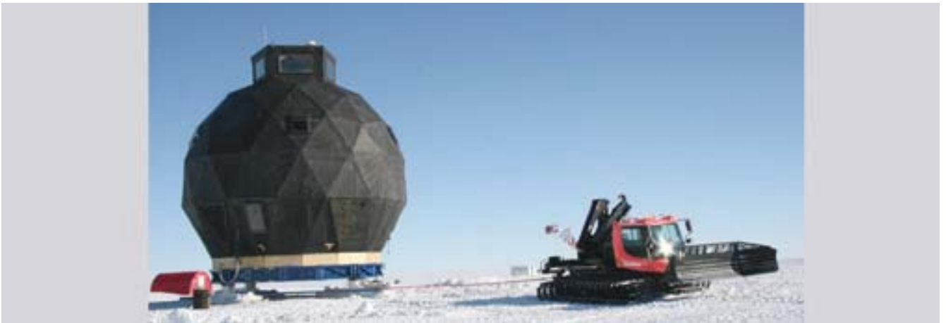
Moving the Dome back to its original position just 4.5 m higher
