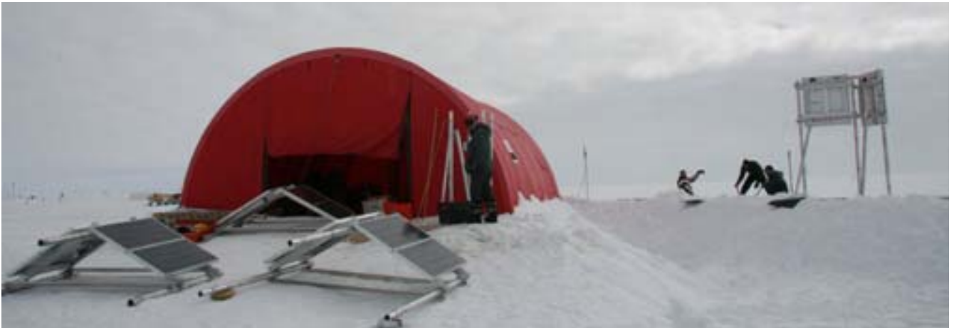
GLISN solarpanel D-frames under construction
